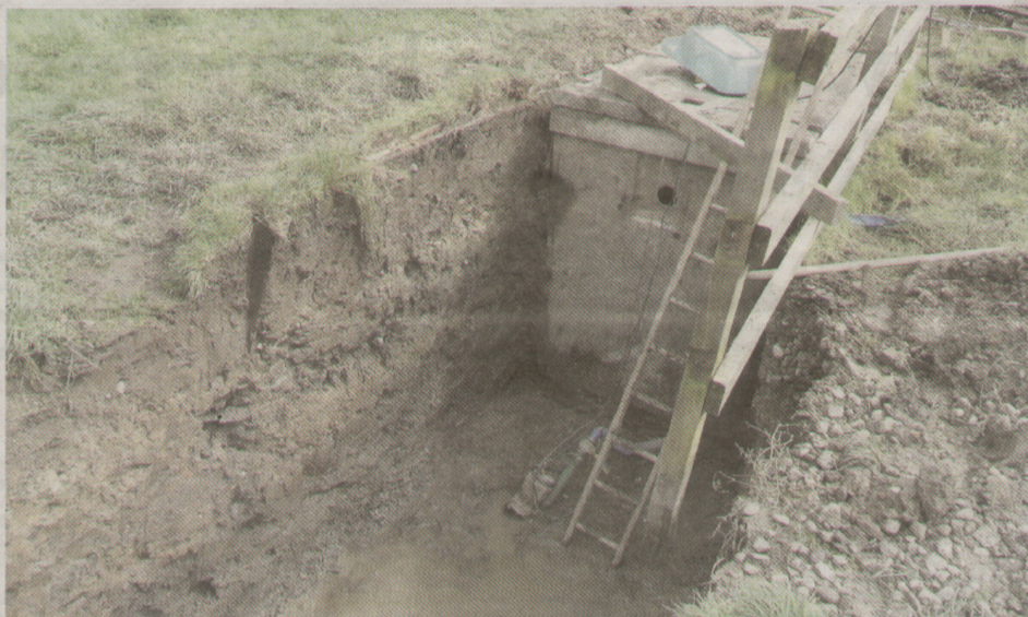
DEVELOPMENTS: Above is a septic tank that is structurally sound but the surrounding soil is tightly packed and contains no gravelly material at all so there is limited soakage. After 10-12 years, the percolation area failed. The solution from O'Reilly Oakstown Environmental was to add a new tank, right, to allow further processing of the waste and boost the efficiency of the system from 30pc with the first tank to 97-98pc in the new system
